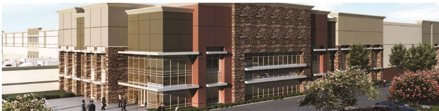
4375 North Perris Boulevard – Perris, CA 1,008,646-square-foot spec industrial building under construction
