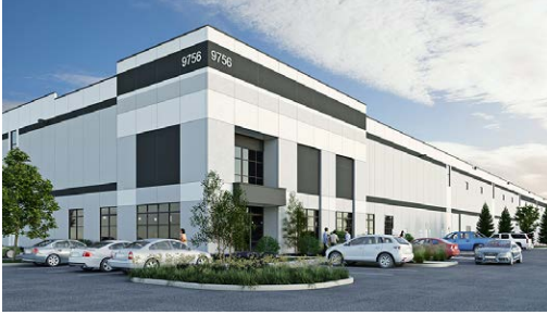
RGLP Intermodal South 9756 – Columbus, OH 574,560-square-foot speculative building with direct rail service via Norfolk Southern
