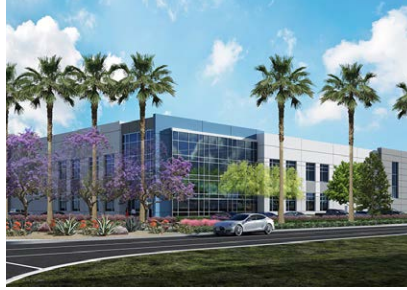
1865 Mountain View Avenue – Redlands, CA 304,262-square-foot speculative building in Inland Empire East submarket
