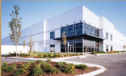
Groveport Commerce Center 437 – Columbus, OH 437,256-square foot new industrial lease
