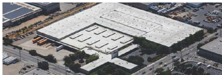
1919 Williams Street – San Leandro, CA 219,000-square-foot logistics building in Northern California East Bay submarket
