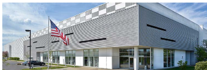
315 Half Acre Road – Cranbury, NJ 650,123-square-foot lease to Cooperfriedman Electric Supply; backfill of a known mid-2020 expiration avoiding any lease-up period downtime
