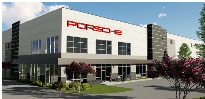
Camp Creek 4850 – Atlanta, GA 210,180-square-foot build-to-suit distribution center for Porsche Cars North America
