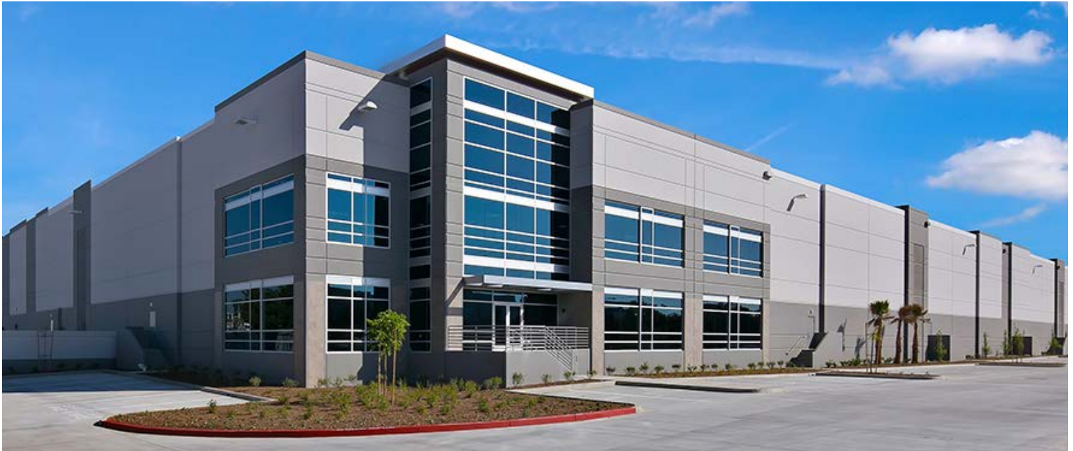
1589 E. 9th Street, Pomona, CA — 197,685-square-foot warehouse that is part of four-building, 751,935-square-foot industrial acquisition in Southern California; 100% leased
