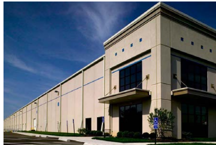
Hebron 2285 – Cincinnati, OH 598,000-square-foot lease renewal with e-commerce company
