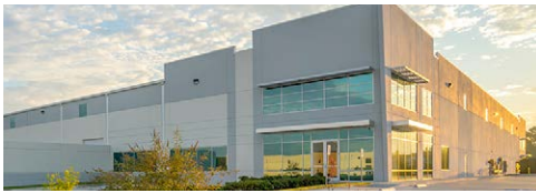
Point North 8221 – Houston, TX 168,850-square-foot new lease with Starplast USA
