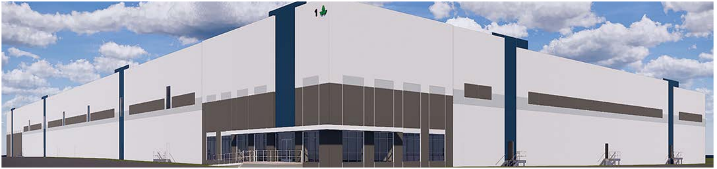
One Paddock Street – Avenel, NJ 185,071-square-foot logistics building; 100% preleased to leading e-commerce company
