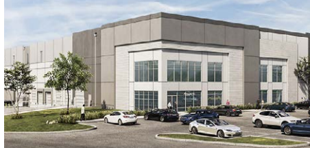
150 Old New Brunswick Road – Piscataway, NJ 622,230-square-foot lease with a national home furnishings retailer
