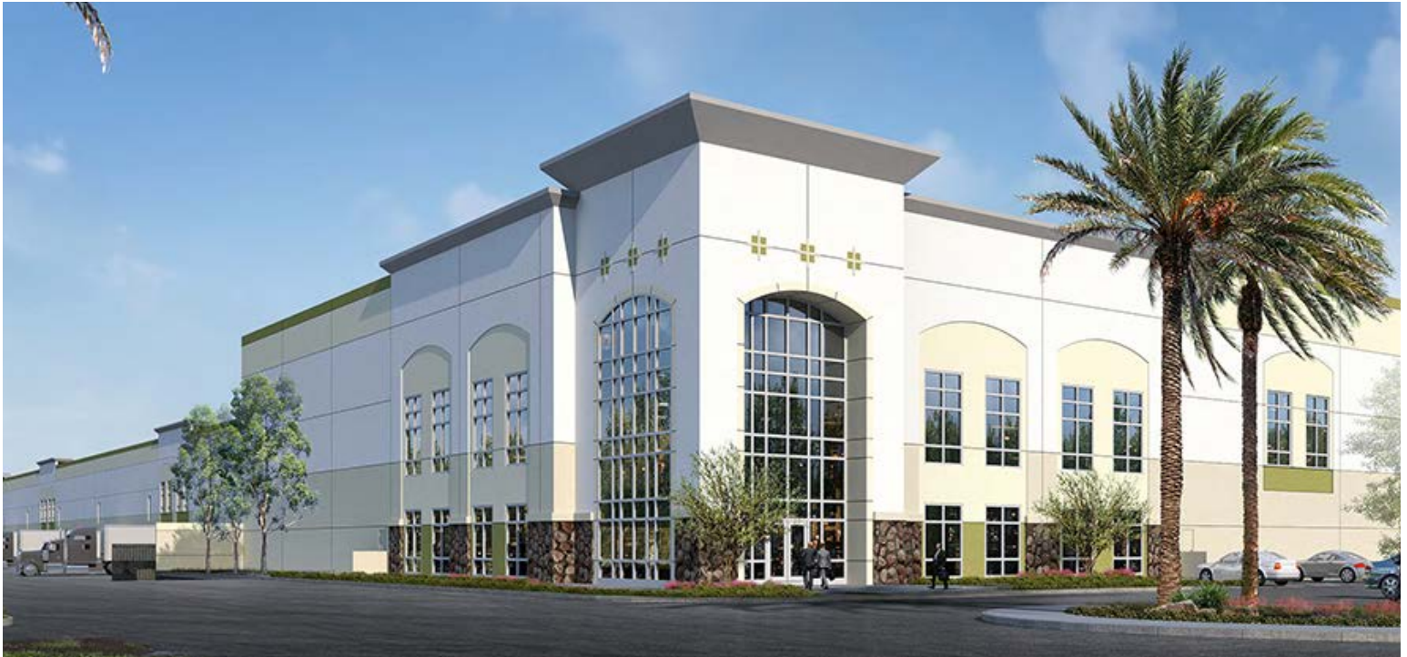
13131 Los Angeles Street, Irwindale, California — 528,710-square-foot, speculative development with enhanced sustainability and smart building features
