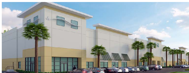
Turnpike Crossing 6711 – West Palm Beach, FL 96,759-square-foot build-to-suit distribution center
