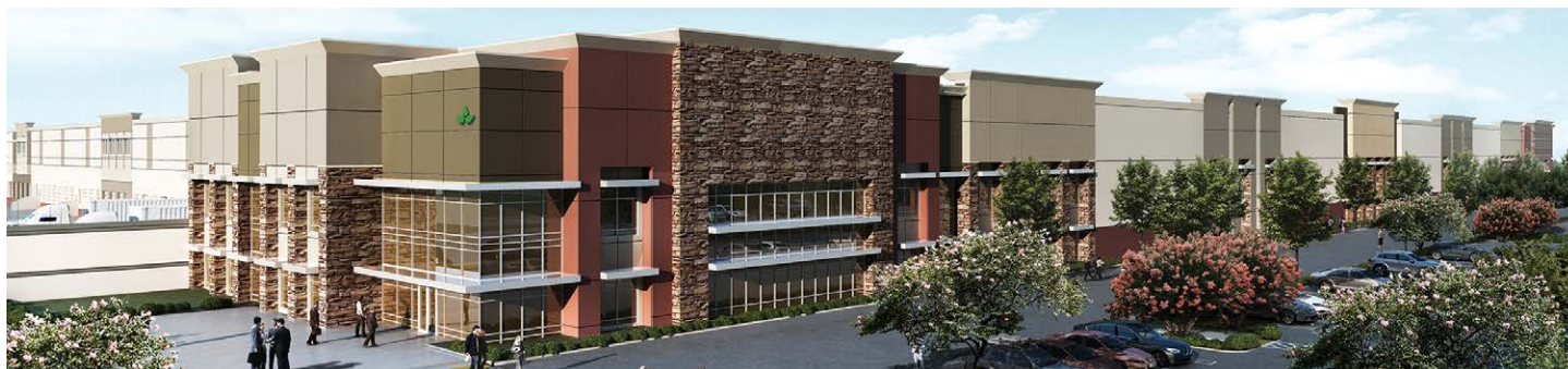
4375 North Perris Boulevard – Perris, CA 1,009,000-square-foot logistics building; 100% leased to leading e-commerce company
