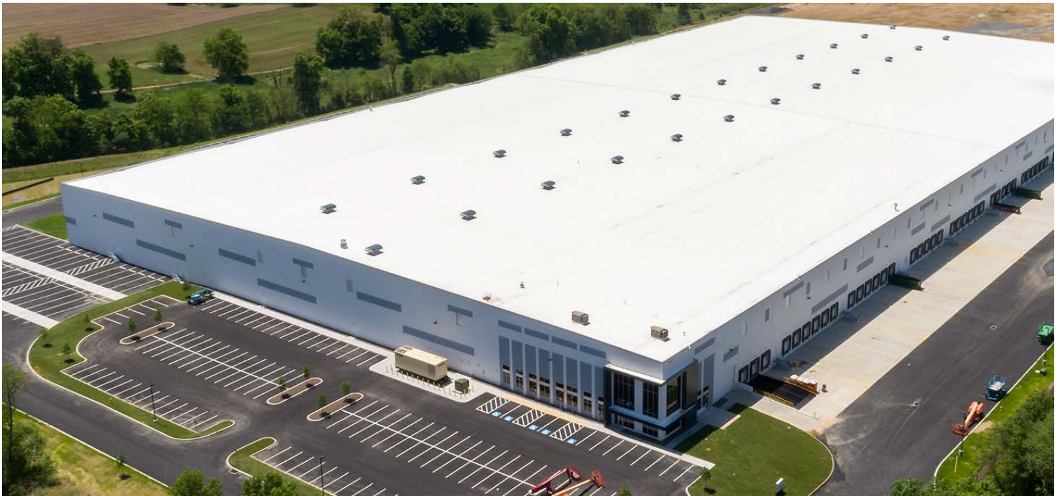
Central Logistics Park 100, Myerstown, Pennsylvania – 616,000-square-foot, build-to-suit logistics center for Max Finkelstein, a regional tire distributor, in the Lehigh Valley
