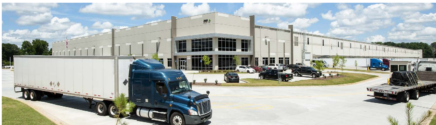
2929 Roosevelt Highway – Atlanta, GA 499,000-square-foot logistics building; 100% leased to a warehouse, distribution and transportation provider
