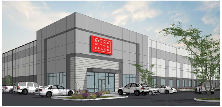
South Afton Industrial Park 3001 – Batavia, OH 617,760-square-foot, build-to-suit distribution center for Design Within Reach
