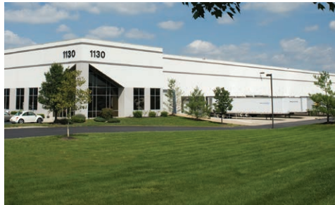
1130 Commerce Boulevard – Logan Township, NJ 215,866-square foot lease with UPS Supply Chain Solutions
