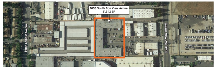
1656 South Bon View Avenue – Ontario, CA 81,542-square-foot facility; 100% leased to one of the largest applicators of powder coatings in Southern California
