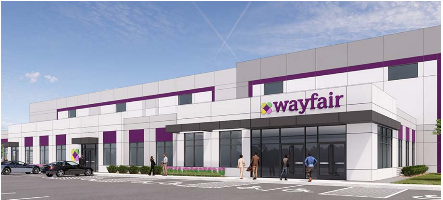
Airport Logistics Center III, Romeoville, Illinois — 1,200,420-square-foot, build-to-suit e-commerce fulfillment center for Wayfair, Inc.
